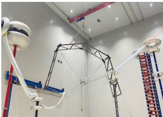
RIV and Visual Corona Test of 345kV suspension string in SHEMAR's Electrical Test Hall
