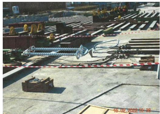
Mechanical Failure Test of 400kV double tension string
